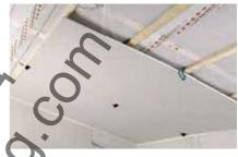
The tools and clamps for convenient, easy and safe installation work on walls, ceilings and especially on inclined areas. The fixing clamps and crosses can be removed are available for other boards, once the board has been fastened with screws.
